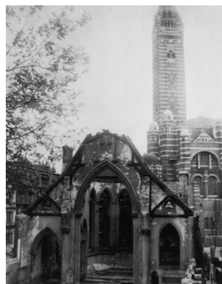
The gutted remains of St Andrew's Church, Ashley Place, after a direct hit in late 1940, showing the proximity of the bomb to the Cathedral.
