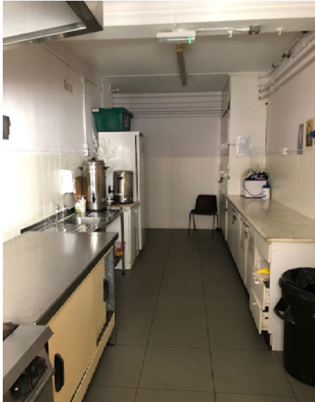
The Kitchen before refurbishment – not an attractive prospect.
