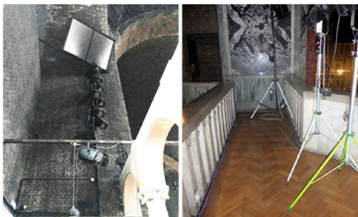
Left: Existing lighting rigs on the back of the chancel arch Right: Loose lighting stands on the transept gallery bridges
