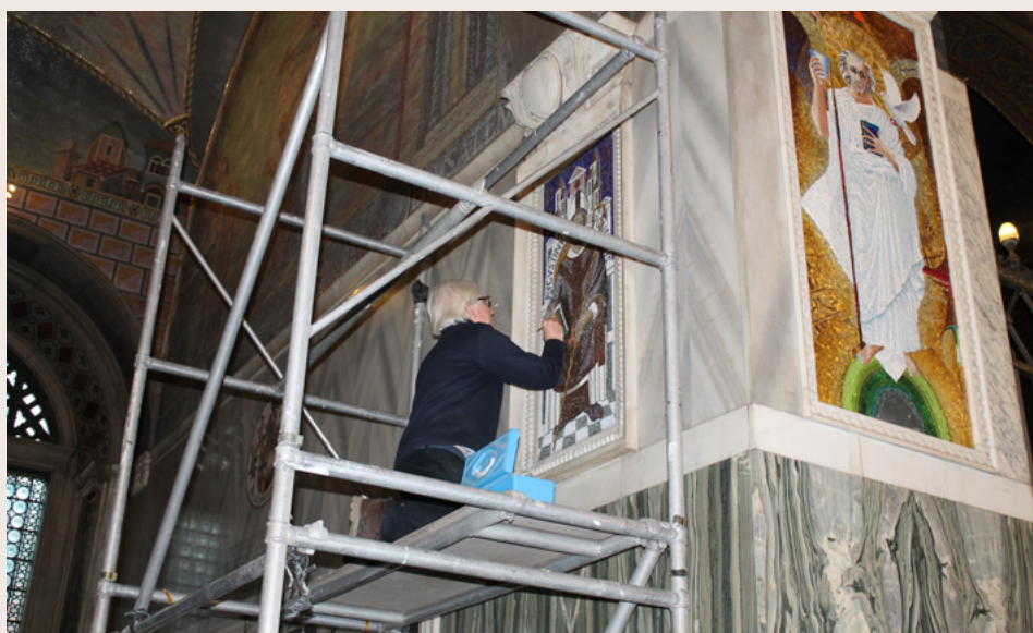
Final touches to the grouting are carried out in situ
