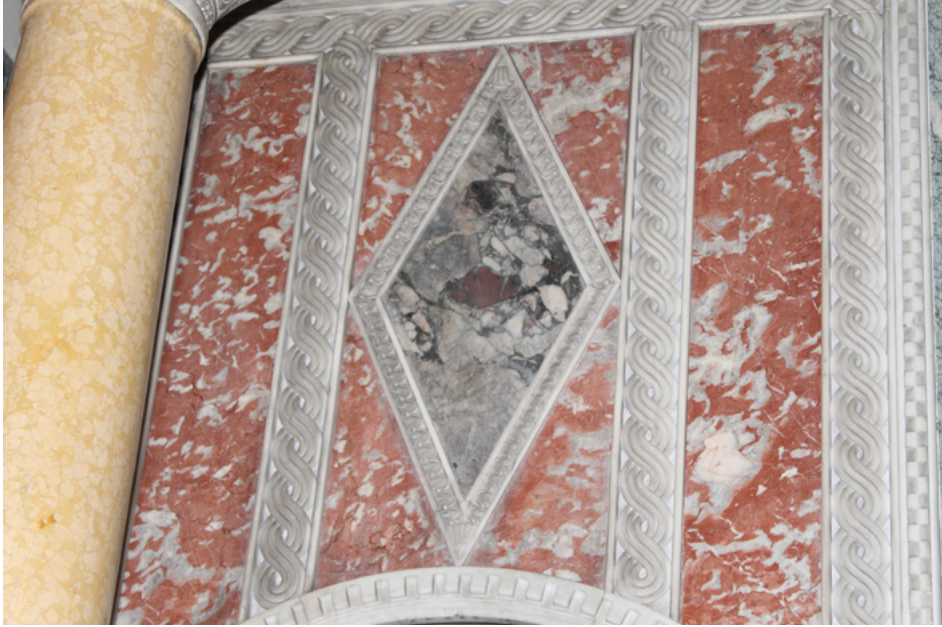
One of two panels of Africano on either side of St Patrick's altar
