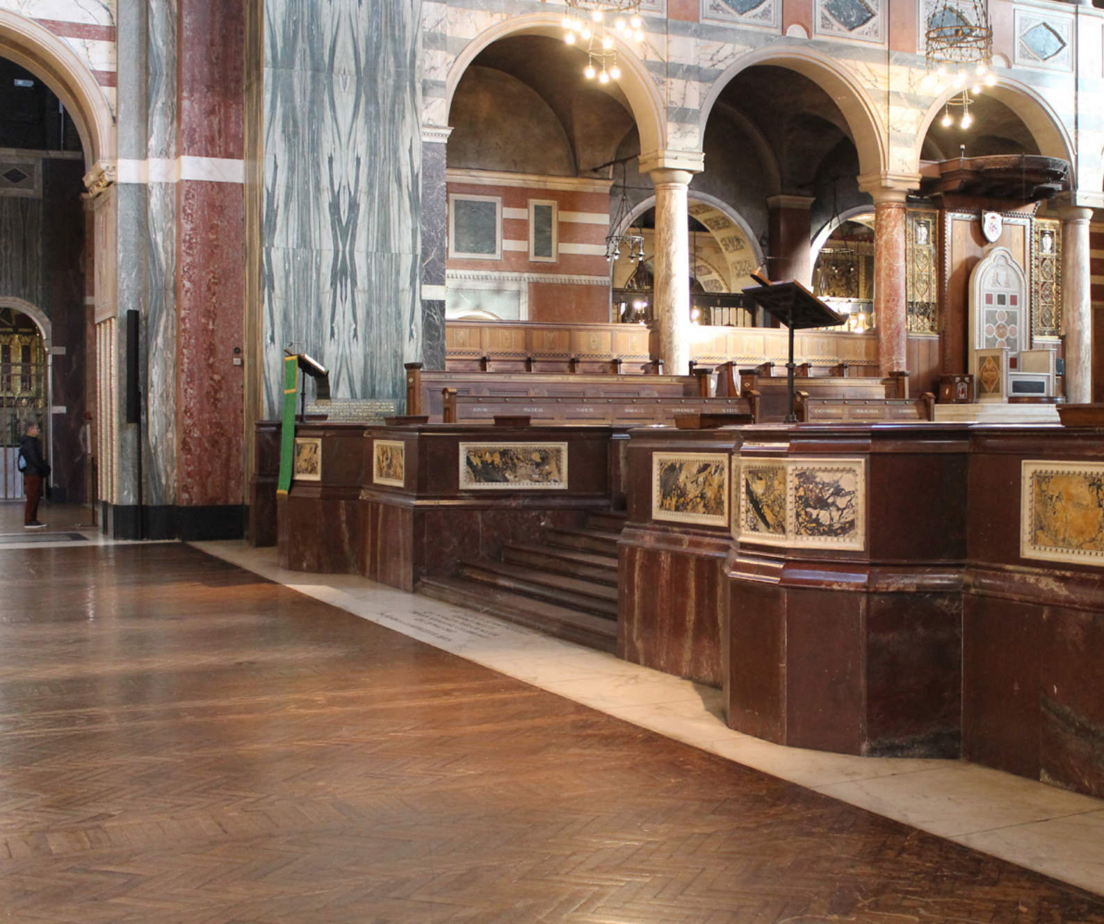
The Balustrade and Sanctuary steps are of Rosso Antico, although the steps are 'scuffed and weathered' by decades of use
