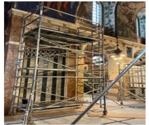
The work requires specialist access
